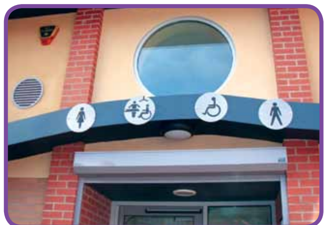
Visually contrasting symbols and non-reflective signage at Newark town centre's public toilet facilities. Opening hours are extended to cater for events
