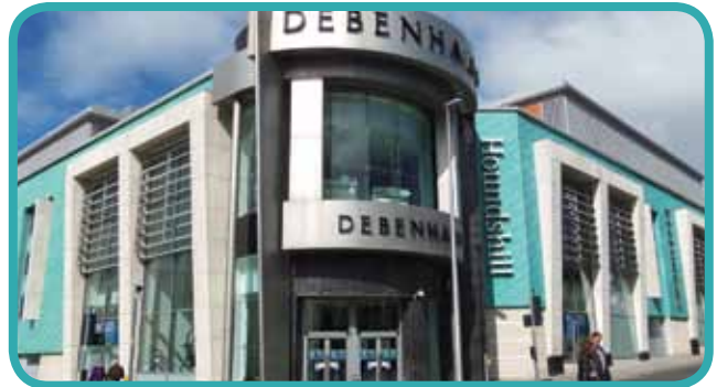
Debenhams Blackpool provided the space for the CP facility, while the council financed the installation and maintenance © John Burke
