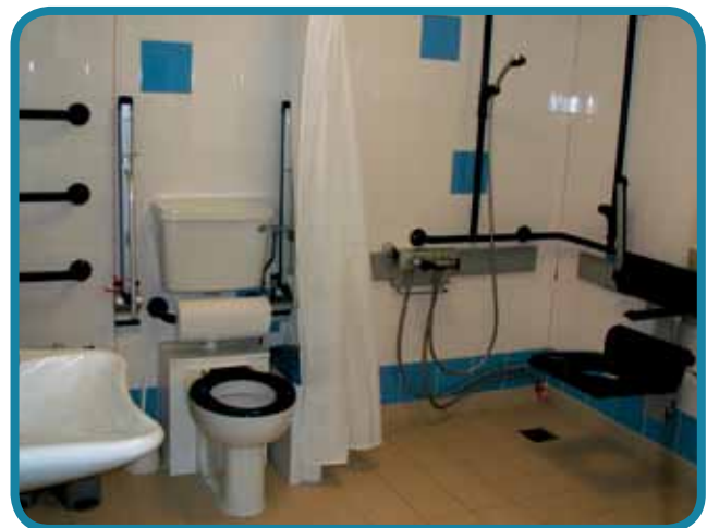
The CP facility at Ken Martin Leisure Centre in Nottingham includes a shower seat with a backrest and drop-down arm supports
